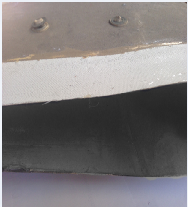
Air supply ducting on a VC-10. Interior is dirty and dusty but has no oil.
